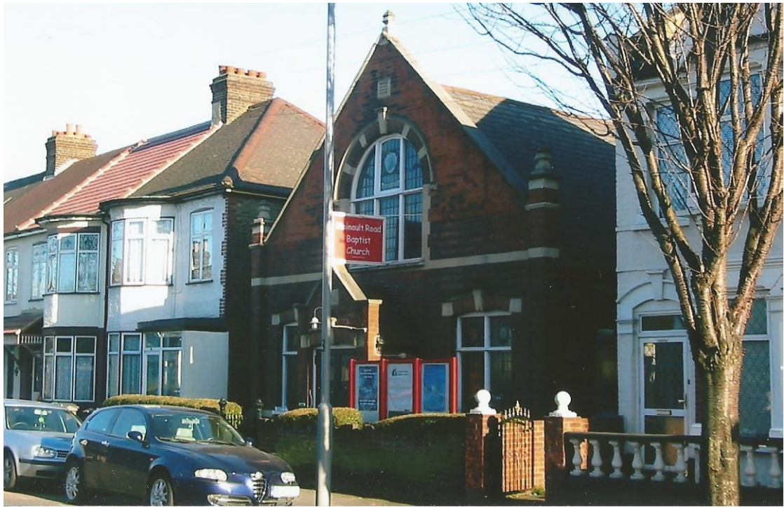
Baptist Chapel, Hainault Road (site of Moyer House) - DIC
